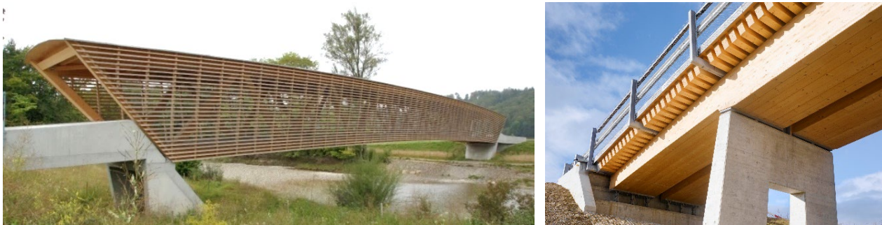
Figure 39: Bridge Neumatt with protected truss system using gladding (left) and Bridge Horen with weather protection by structural overhang
