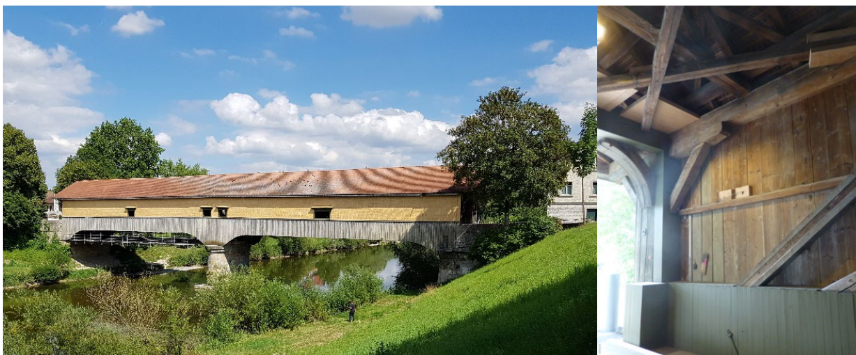
Figure 30: Bridge crossing the Thur in the village of Andelfingen with a view on the instrumentation and two dummy blocks on the north side of the bridge
